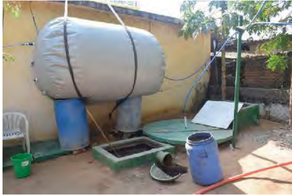
Fig 2: Solid Waste management facility in the adopted village
